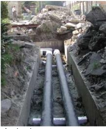
Photo 8. Installing new district heating pipes
